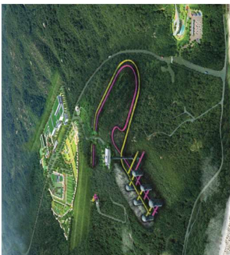
Underground Silo Disposal Facility
