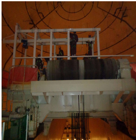
Install Rigging Frame
