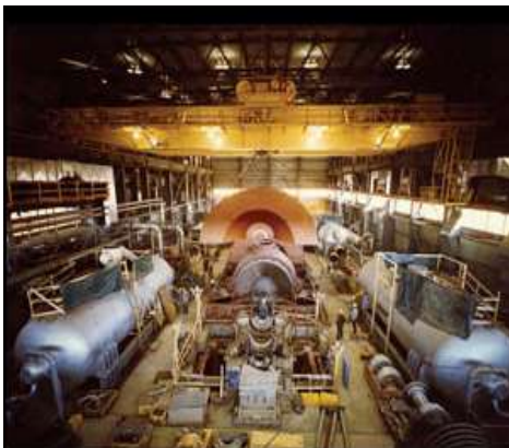
← Turbine Building under LP Rotor maintenance
