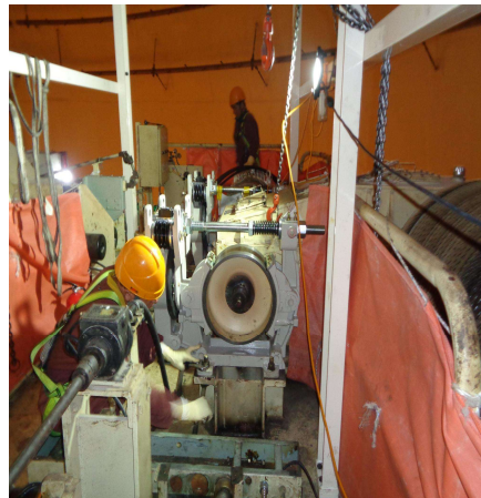
Install Main Hoist Brake
