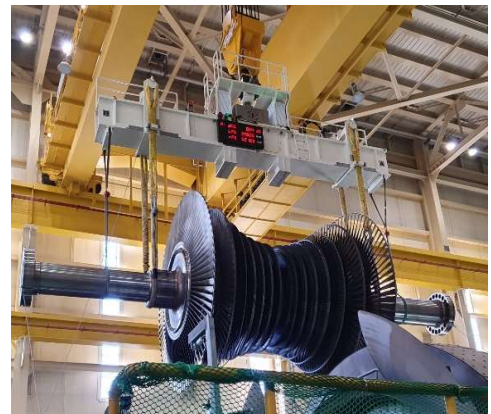
← Turbine Building under LP Rotor maintenance
