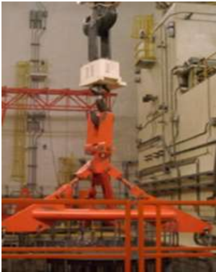
← RV Internal hanged by Polar Crane with PLP
