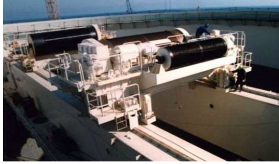
Emergency Brake and Failure Brake of COSAS installed at Hoisting Device of Polar Crane
